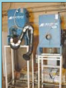
(10) Air-Flow Systems Inc. Flex Arm Type Mist Collectors
